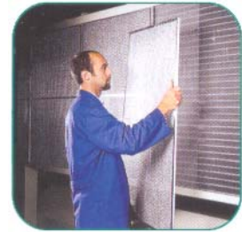
Filtermatten am Kondensator Condenser air filters
